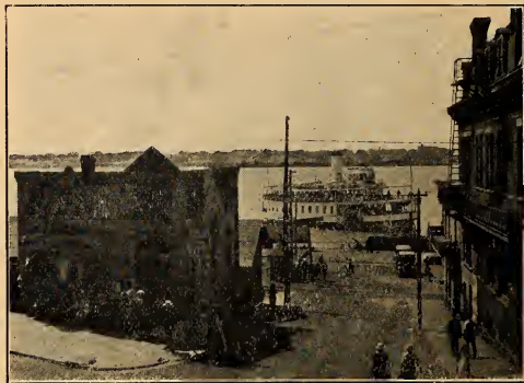
FERRY WHARF, SARNIA.
